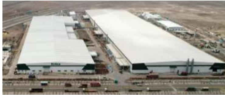
Dholera module plant (2.4 GW)
