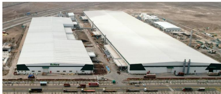
Dholera module plant (2.4 GW)
