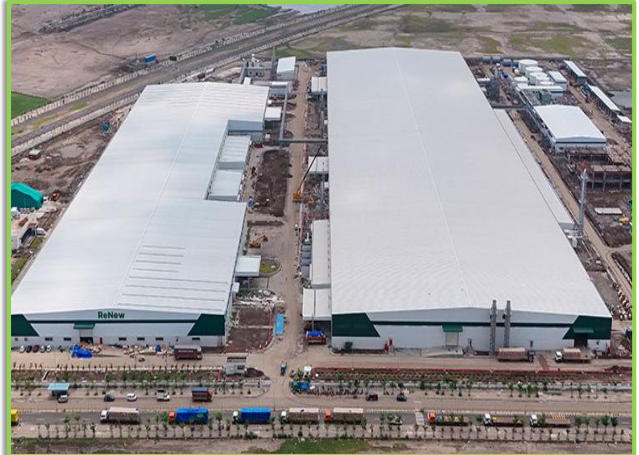
ReNew's manufacturing facility in Dholera, Gujarat
