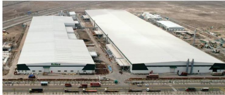
Dholera module plant (2.4 GW)
